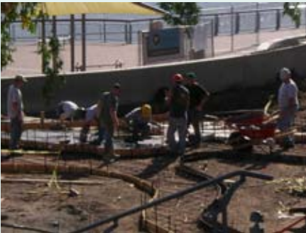
Pouring Lake Winnipeg - Summer 2008
