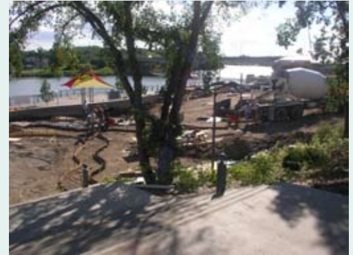
Pouring Lake Winnipeg - Summer 2008
